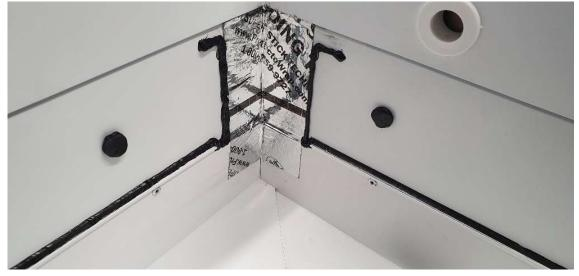
6.1.5 Add sealant to inside of covers just below the top as shown.
