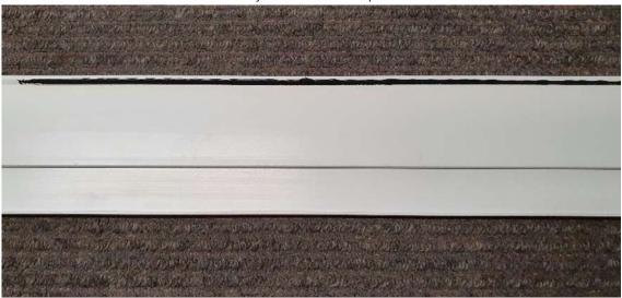
6.1.6 Install covers ensuring they are pushed up hard into the beam incision. Secure with  $1/8^{th}$  rivets 100mm from each corner and evenly spaced at max 3.0m centers.
