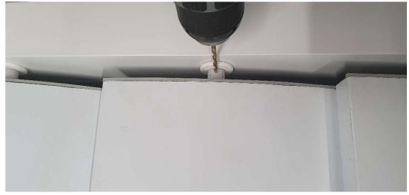
10.1.4 Using a 3.0mm drill bit, drill out every second blade's idler end spigot approximately2.0mm away from the flange of the corresponding bush.
